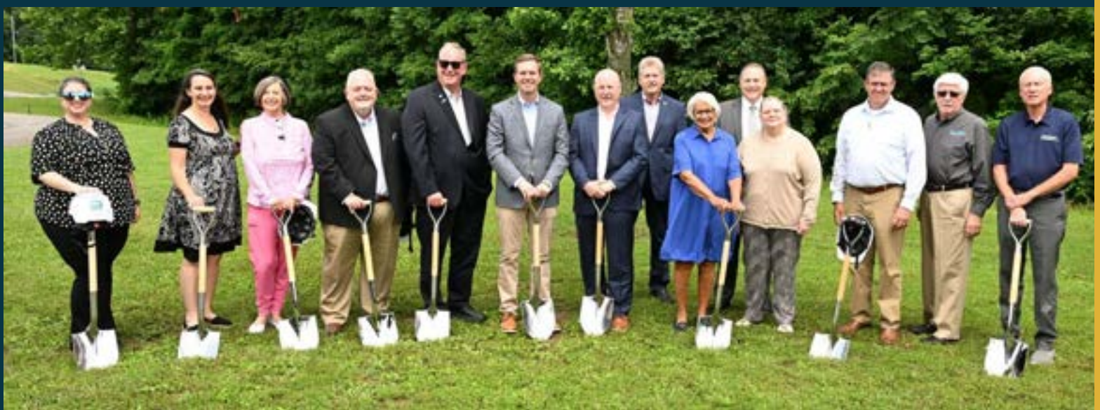
Governor Andy Beshear helps members of MEGA's Board of Directors and the Foundation's Advisory Council celebrate the groundbreaking for BE&E, the first manufacturing facility to be built at Paradise Regional Industrial Park.
